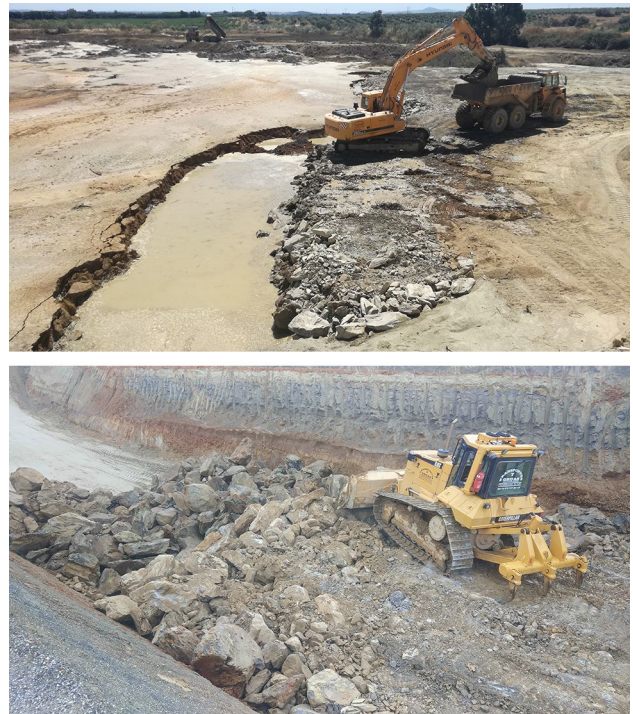
Figs. 11 and 12 Tailings removal and replacement with coarse selected material
