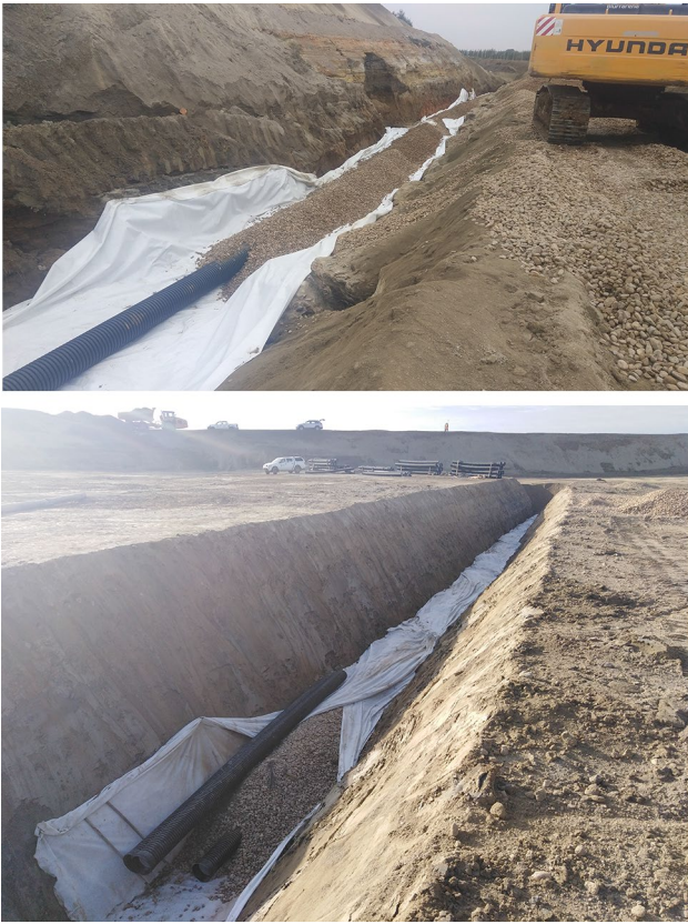
Figs. 13 and 14 Installation of the sub-drainage system
