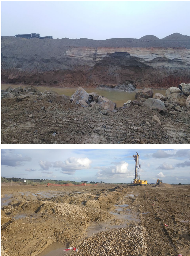
Figs. 9 and 10 Left: excavation and substitution of old tailings. Right: execution of the gravel columns
